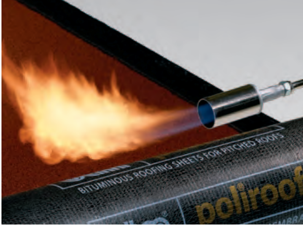
BTM Poliroof PR 4500 (propane torch applied)
